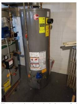
Water heater is estimated to be between 3 - 12 years old. Water heaters have a typical life span of 8 - 12 years.
