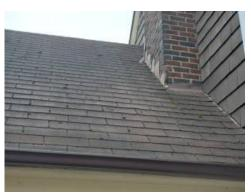
Roof penetrations represent a weak link in any roof. Flashings or seals should be monitored for deterioration caused by age and exposure, and repaired as required. Chimney flashings should be cut-in to the mortar prior to caulking.
